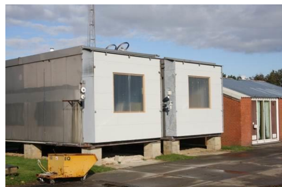
Figure 10 – Test Cell at BBRI
